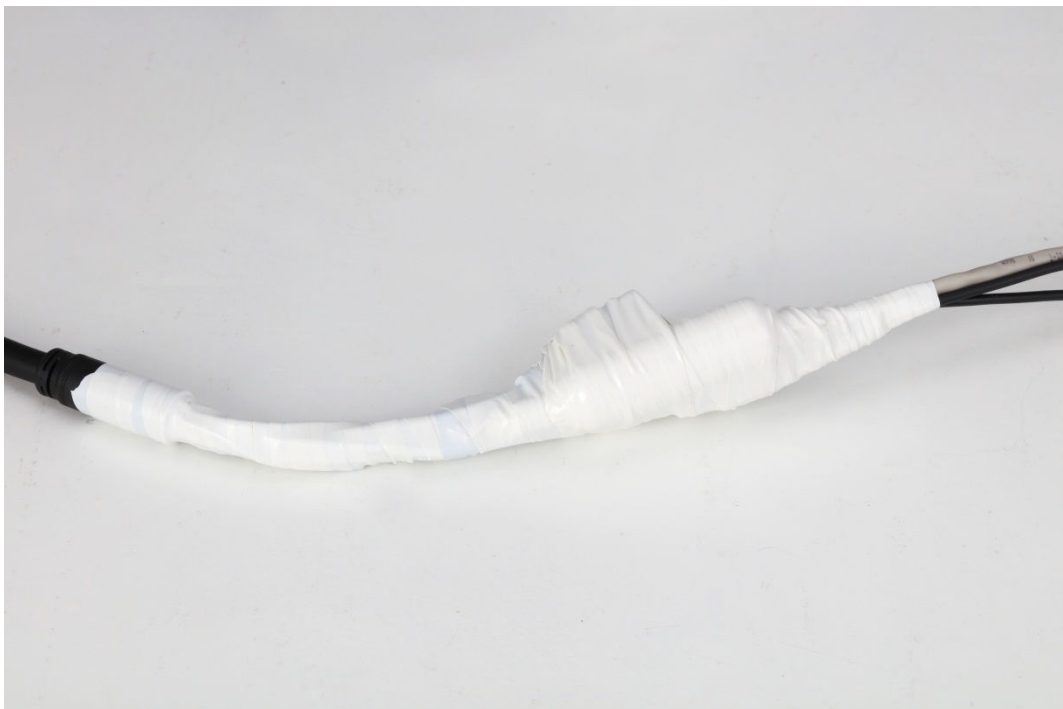
Figure 1-3 Covering exposed parts
